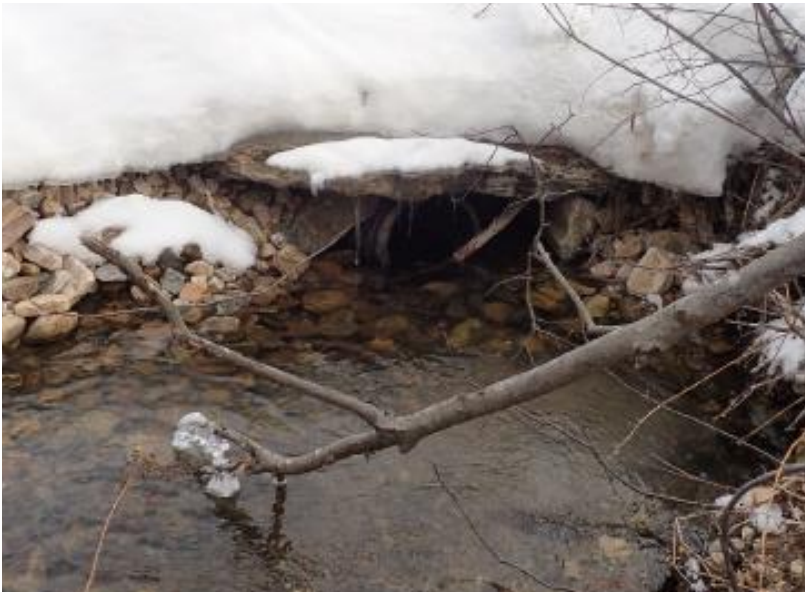
Figure 3.6: Partially Collapsed Culvert under Frost Road at Savery Brook
